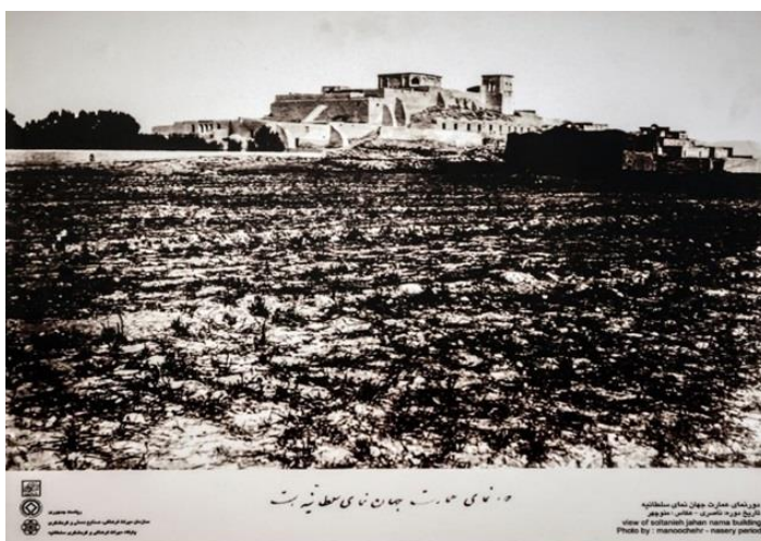
Fig. 11. The Qajar palace at Sultānīyya with an adjacent structure. Photograph from the local archive of the Iranian Cultural Heritage, Handicrafts and Tourism Organization (ICHTO), Sultānīyya World Heritage Site.
