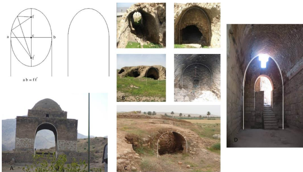
Fig. 8. Tond mazey arches in the four-iwan of Niasar, ruins of Qal'eh Hazaar in Dareh Shahr, ruins of the Khosrow building in Qasr-e Shirin, and the Palace of Khosrow in the Fire Temple of Shiz in Takab (by the Authors).
