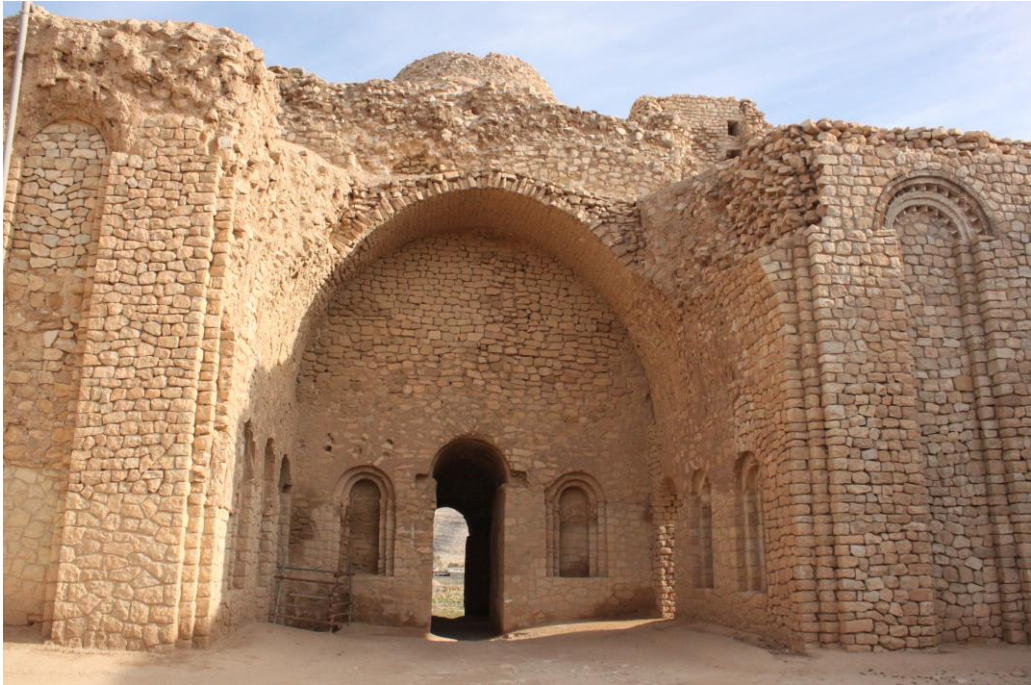
Fig. 1. Entrance iwans of the Palace of Ardashir with semi-circular arches in Firuzabad, Fars (by the Authors).
