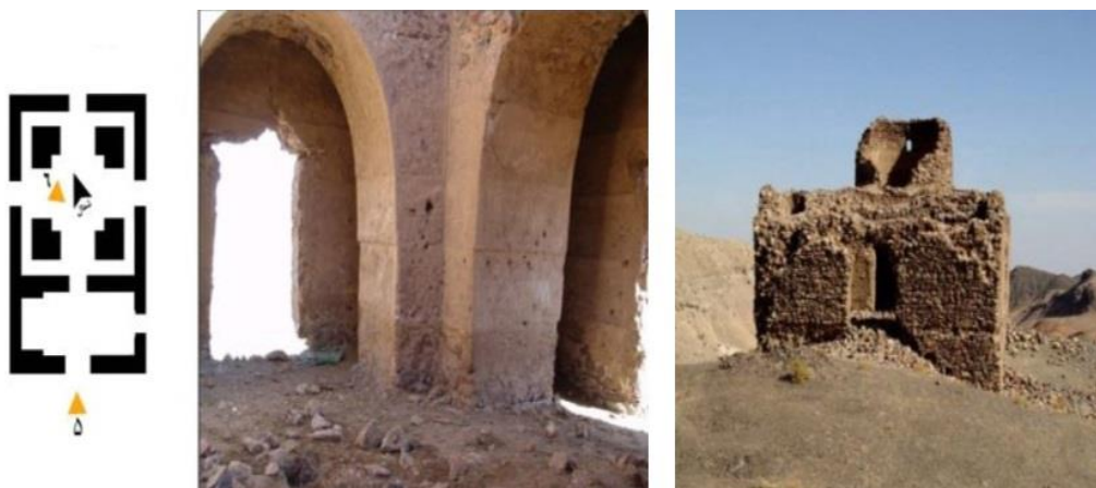
Fig. 2. Four-Iwan of Negar with semi-circular arches in Kerman province (by the Authors).
