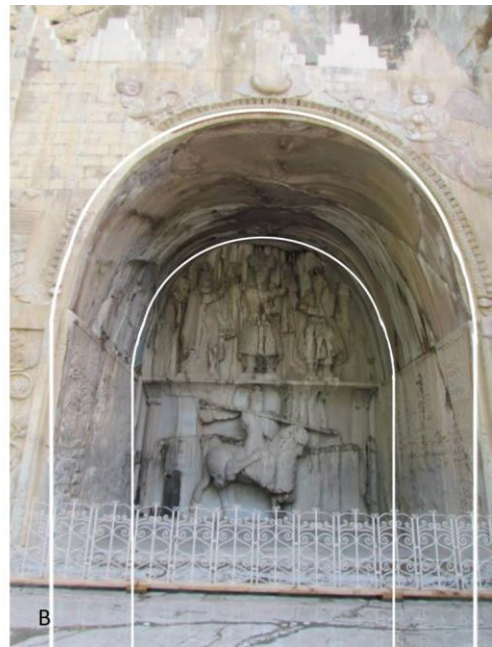
Fig. 10. Slow mazey arch in the Palace of Ardashir in Firuzabad and Taq Khosrow in Taq-e Bostan, Kermanshah (by the Authors).
