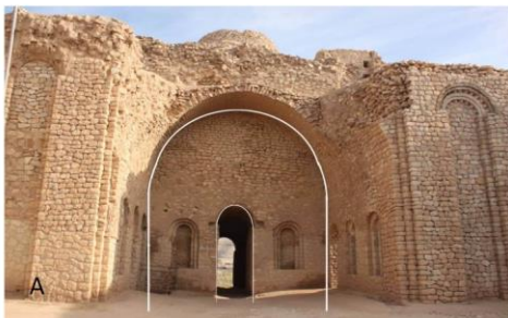
Fig. 10. Slow mazey arch in the Palace of Ardashir in Firuzabad and Taq Khosrow in Taq-e Bostan, Kermanshah (by the Authors).
